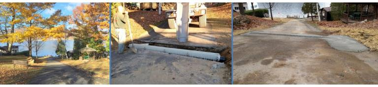
Trench drain to divert water to dry wells before (left), during (middle), and after (right).
